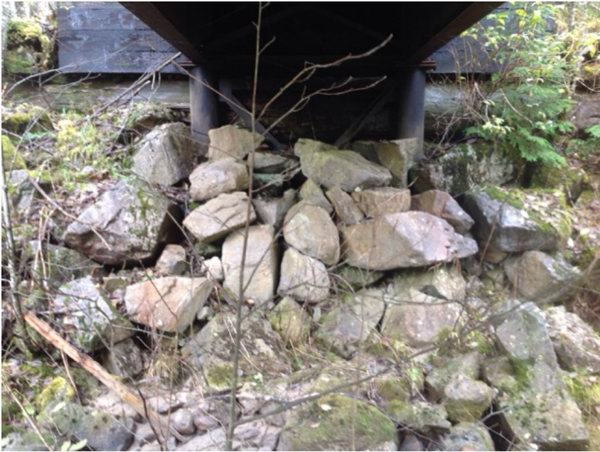
Left Bank Abutment when facing downstream
