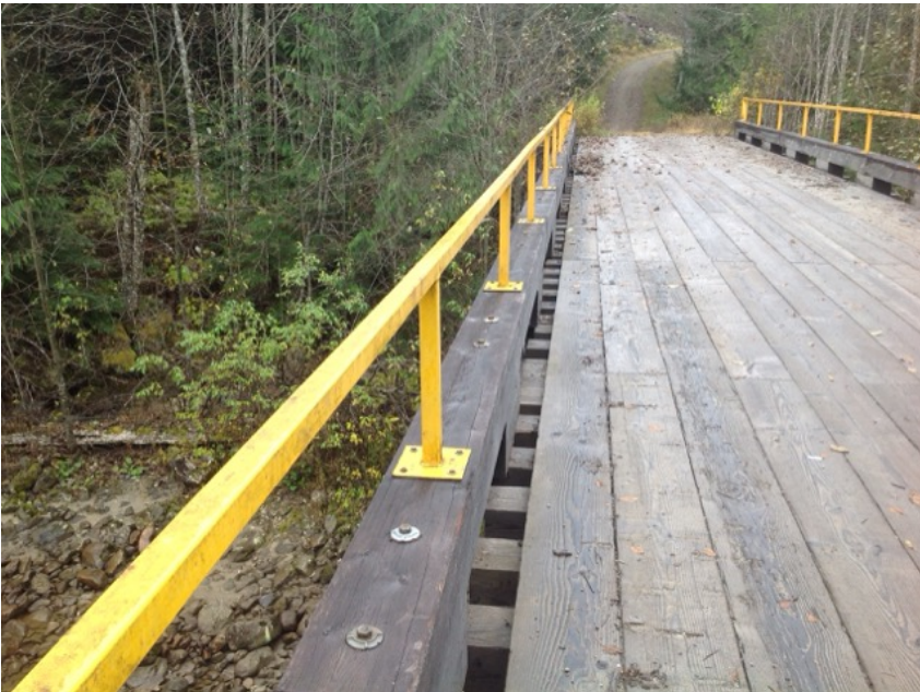
50mm x 50mm HSS handrail
