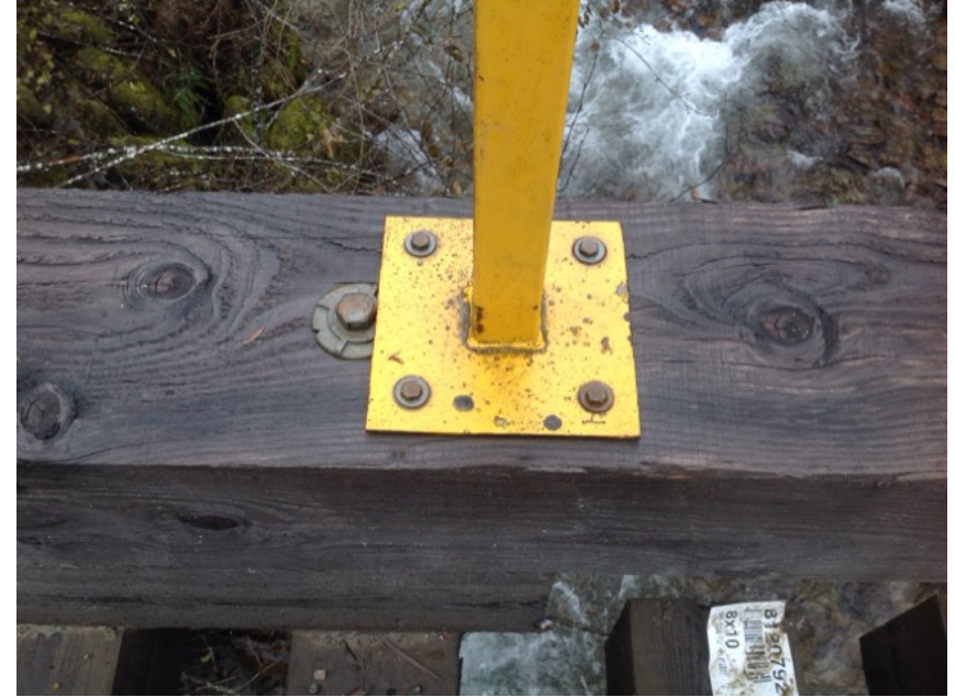
handrail connection to curb
