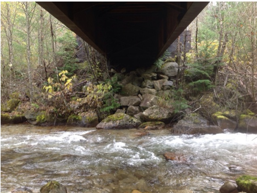
Right Bank Abutment when facing downstream
